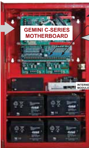
GEMC-BSLC Burg SLC Mod. and GEMC-FW-SLC Fire SCL Mod Mount beneath motherboard
